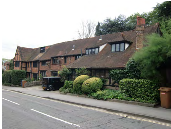
Picture 3.37 Good grouping of the Tithe Barn, Stanmere House and Old Church House on Old Church Lane
