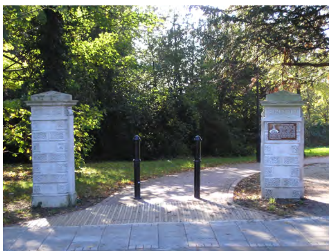
Picture 3.57 Grade II Listed entrance piers to Stanmore Park
