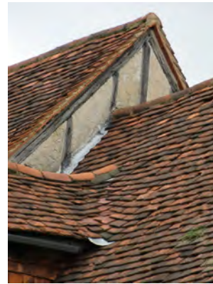
Picture 3.65 Varied roofscape and timber framing and render panels on Church House Cottage, Old Church Lane
