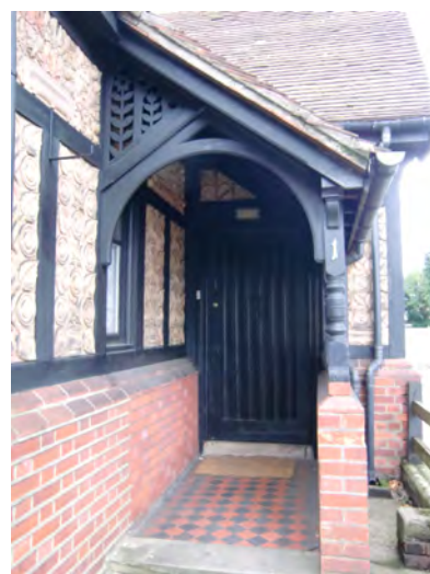
Picture 3.41 Good timber framing and decorative timber porch detail
