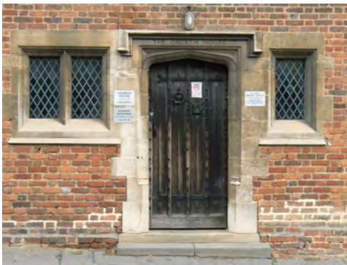
Picture 3.66 Stone and timber Tudor revival style details to the windows and door of Church House, Old Church Lane
