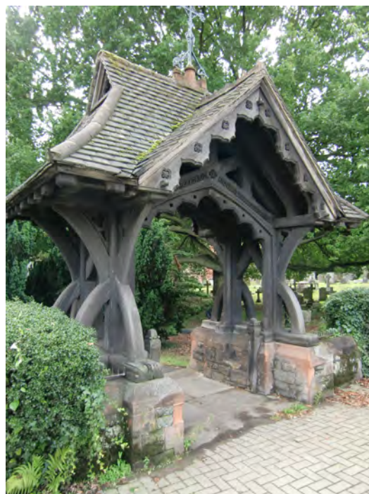
Picture 3.55 Grade II* curtilage listed lych gate to St John the Evangelist Church, Uxbridge Road
