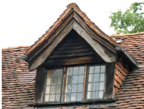
Picture 3.68 Small pitched roof dormer on Church House Cottage, Old Church Lane
