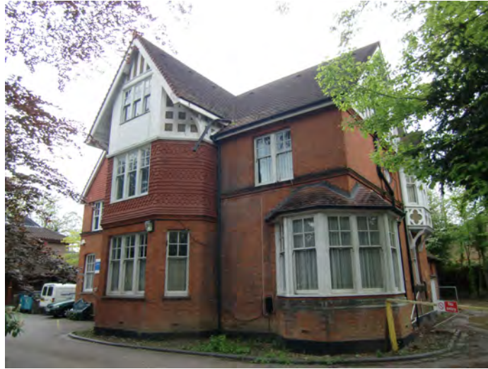
Picture 3.21 Orme Lodge, junction of Gordon Avenue and Old Church Lane
