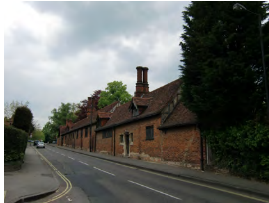
Picture 3.50 Grade II listed Cowmans Cottage, Church House Cottage and The Church House
