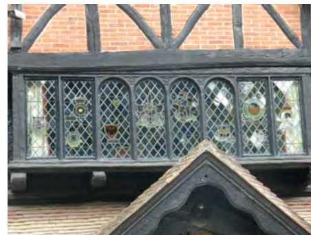
Picture 3.46 Stained glass detail to the leaded light oriel window with delicately carved timber work around it
