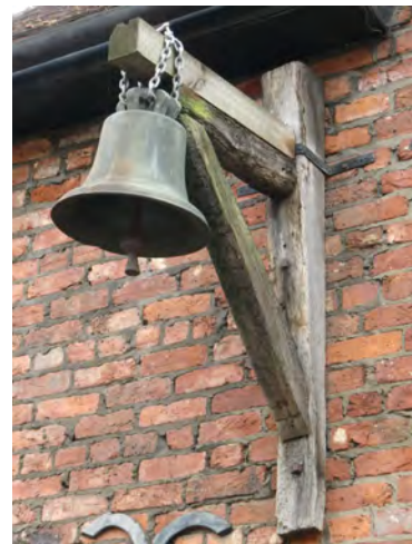
Picture 3.73 Bell on the Grade II listed Tithe Barn
