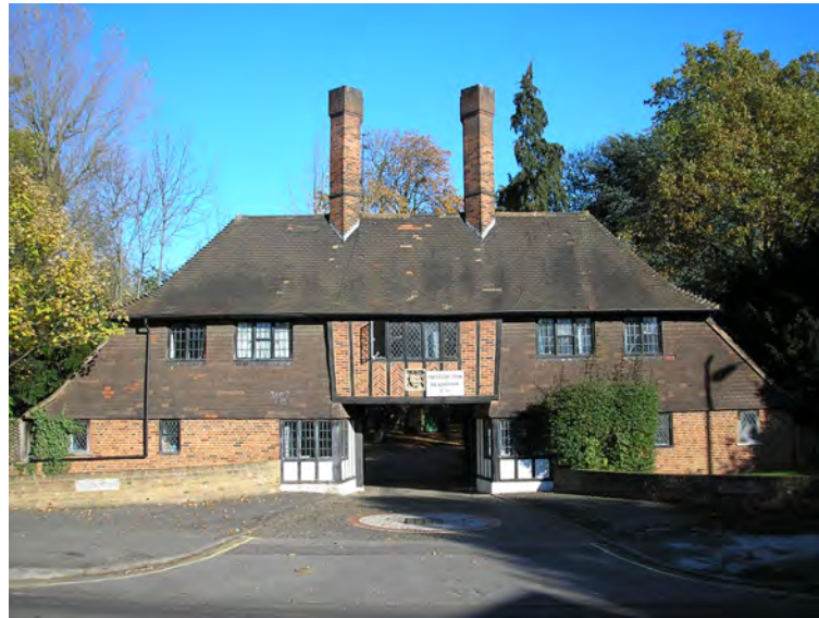
Picture 3.47 Locally listed Tudorbethan Gate House Lodge, Old Church Lane
